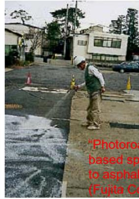
"Photoroad" cement-based spray coating to asphalt paved road (Fujita Corp.)
